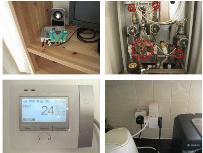
Fig. 5. Examples of home network components deployed in the prototype installation. Starting clockwise from the top left corner, they depict a UWB platform measuring occupancy, an Xbee sensor monitoring the boiler operation, a Zigbee HA plug module and a Zigbee HA Thermostat.
