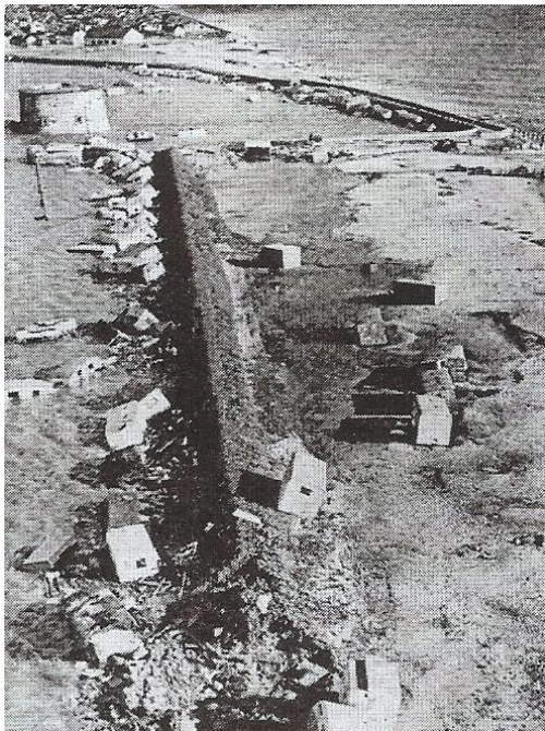
Figures 17 a) & b): the area along the sea defences between Saint Osyth Beach and Jaywick at the new Tower Caravan Site: a) before, and b) after the flood. The Martello Tower at Jaywick can be clearly seen in each photograph.
