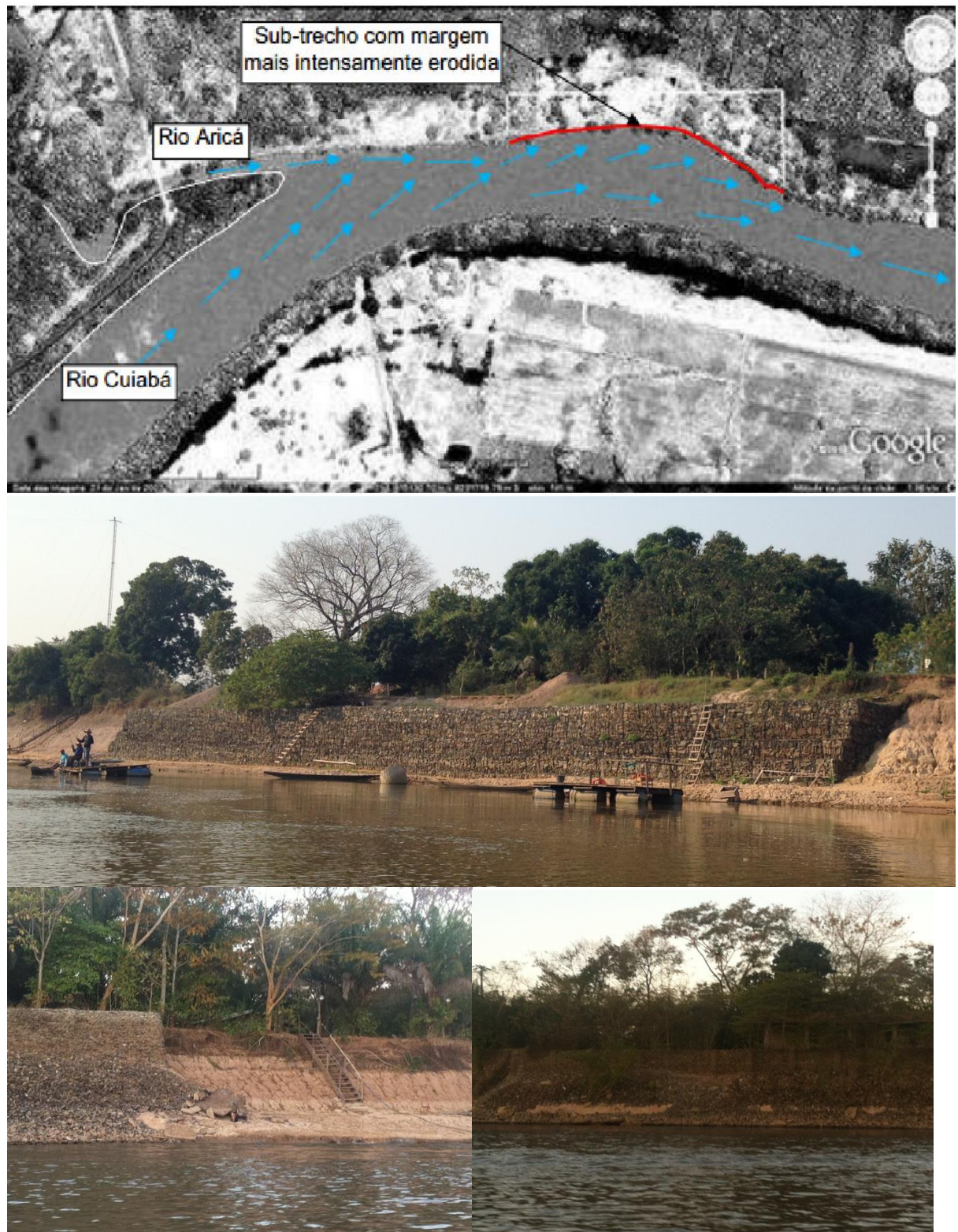
Figure 22: From top to bottom: Diagram from Ximenes de Tavares Salmao et al. (2011) showing erosion in Pesquisa Florida at the confluence of the River Arica and River Cuiabá. Photo of Gabion in eroded area in 2014. Two bottom photos show the collapsed Gabion in 2015.
