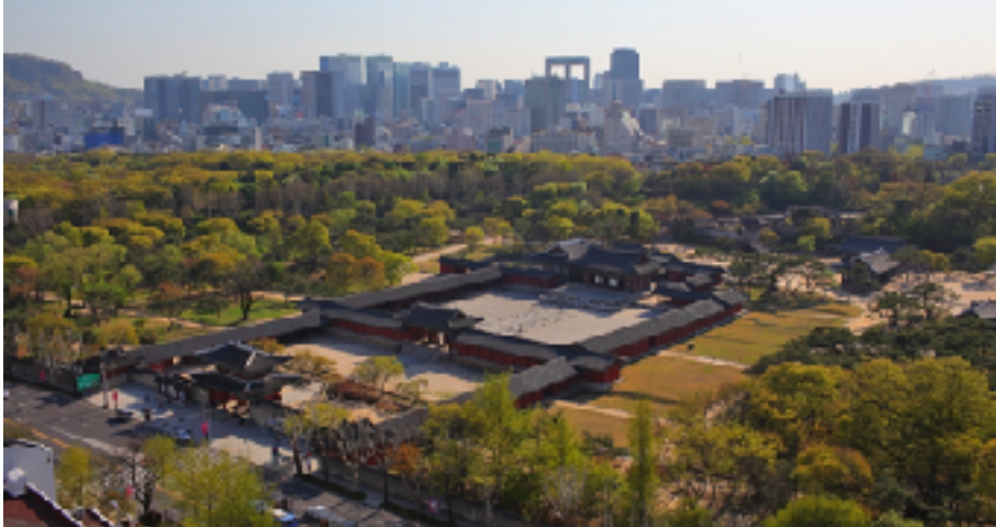
Image 19. Changgyeonggung Palace Complex in 2015 Source : Seoul City website (2015)
