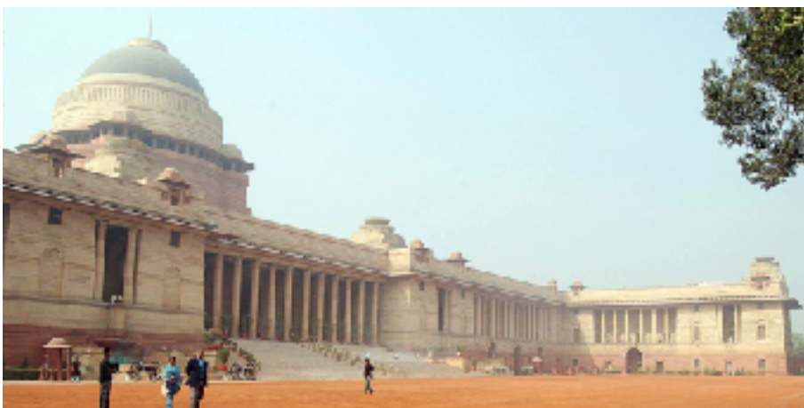
Image 30. (upper) The Japanese Governor-General building (Seoul, 1950s). (below) The British Governor-General's building (New Delhi, 2014). The Japanese Governor-General building was influenced by The British Governor-General's building. Source : Wikipedia ( 2014)
