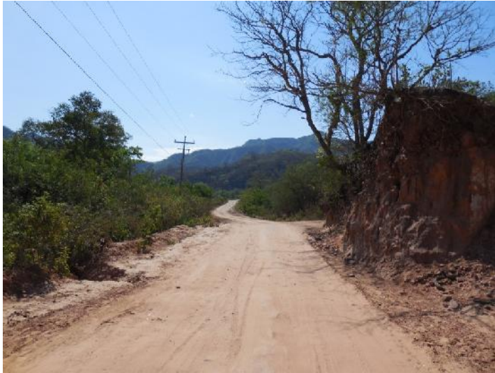
Photo 34 Long Road connecting all Houses in Mandiyuti
