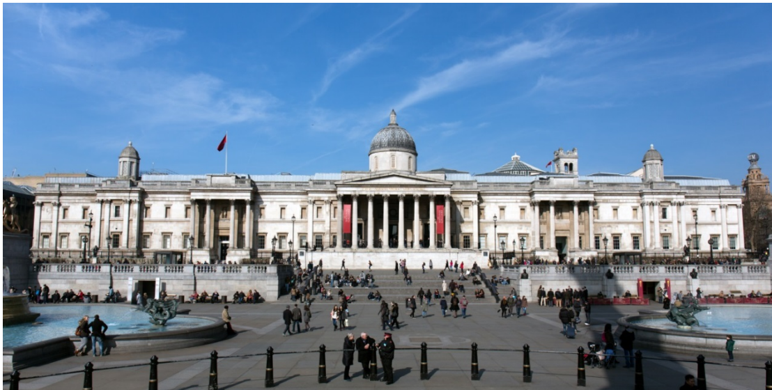
Figure 1b Façade of the Wilkins building
