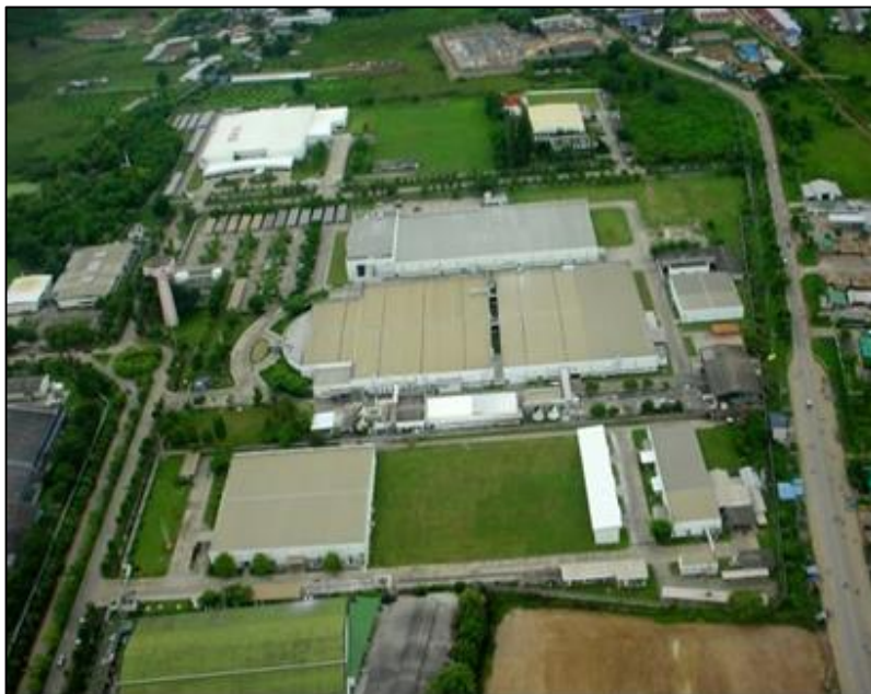
Figure 2.4 The factories around the eastern side of the superhighway
