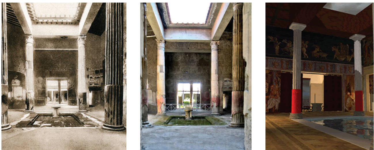
Figure 2.4. Corinthian atrium of villa delle Nozze d'Argento, Pompeii. Left: restoration of the 30s. Centre: restoration of the 60s. Right: virtual restoration by C. Fabius.
