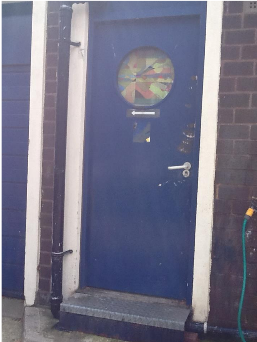
Fig. 7.4 The boiler room/kit storage (Sid)
