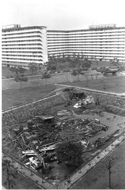
(Fig. 4. Three images of a temple in Toa Payoh, as HDB flats go up in 1968, as seen in 1971, and then as demolished in 1977.)
