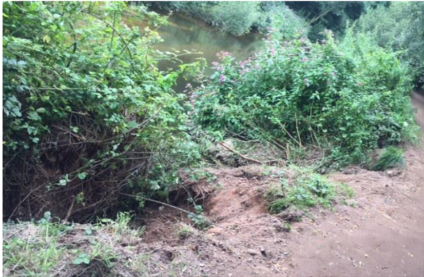
Plate 17. Erosion, Poor Bankside Stability (Frampton, 2017).
