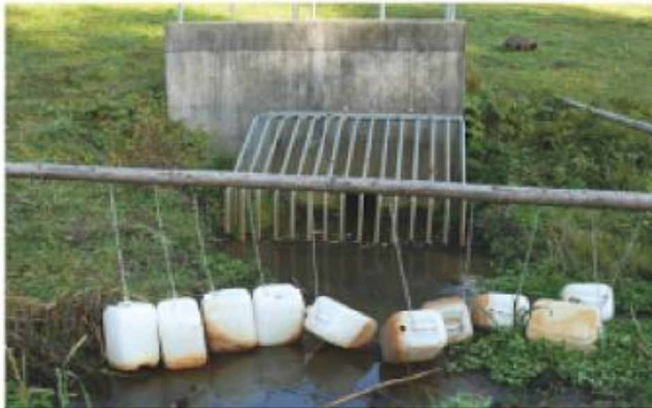
Plate 4. Drainage Culvert Beaver Mitigation (Schwab, G., cited in: Campbell-Palmer et al. , 2016). Some culverts can act as damming points and removal of debris by humans can be effective but time consuming, as well as the knowledge that beavers having a persistence, will possibly return to continue dam construction. Therefore mitigation is focused on making the area surrounding a culvert appear unattractive to beavers. Plate 4 is a mitigation measure designed to hinder the transportation of woody material by Castor fiber to the culvert (Campbell-Palmer et al. , 2016).
