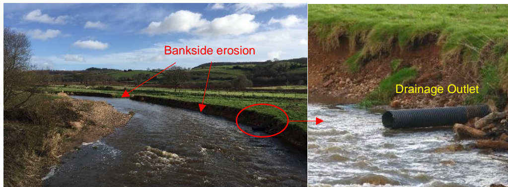
Plate 23. Drainage Outlet Through Eroding Bankside (Frampton, 2017). This stretch of river appears to be important for agricultural land drainage, with high valley sides. However, this may be contributing to erosion of banksides due to excessive water levels and flow rates in wetter months.
