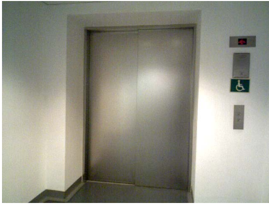
(a) Elevator when the door is closed.
