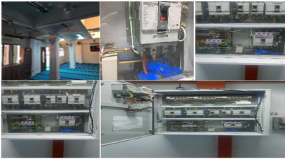
Figure 3: Installation of our energy monitoring system.
