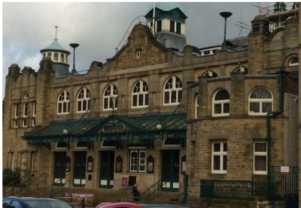
Figure 188 Photographic view of the exterior of the Royal Hall, Harrogate, Yorkshire Source: Cannell, 2017
