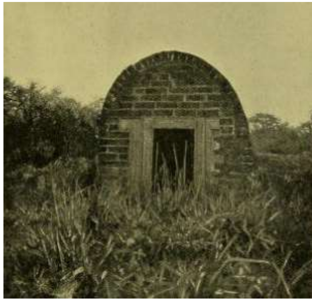
Figure 280 Photograph of the South Weald well head 1907 Source: Christy and Thresh, 1910.
