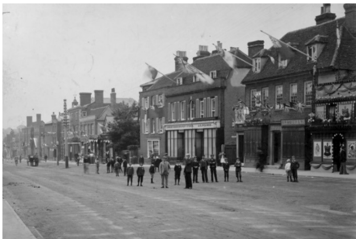
Figure 377 Photograph of Newland Street, Witham showing the Georgian facades of many buildings Source: Gyford, 2005
