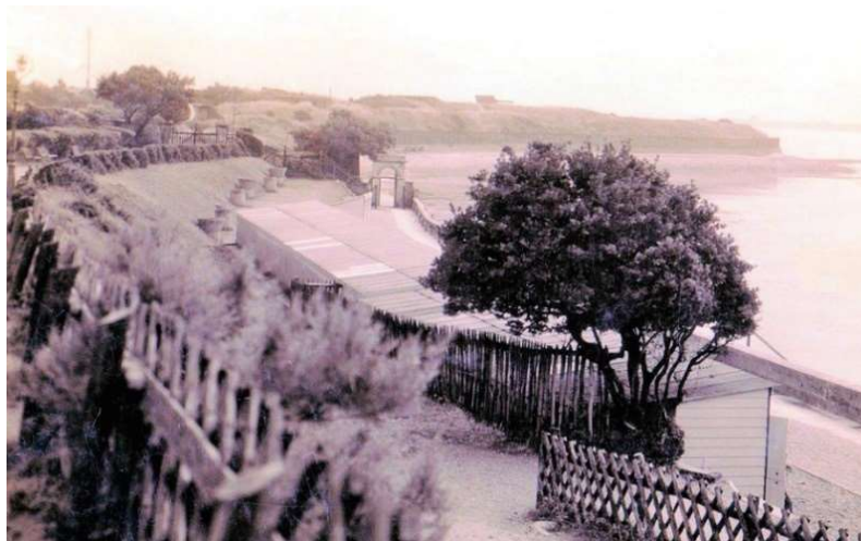
Figure 128 Photograph of the spa site following demolition, circa 1920 Source: Harwichanddovercourt.com, 2017.
