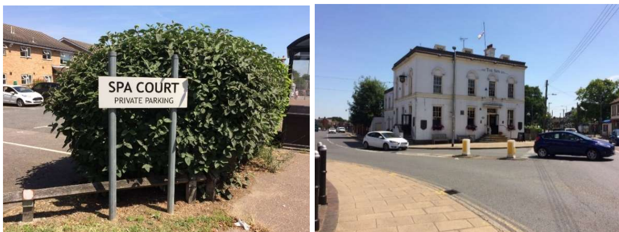
Figure 205 Photographs showing Spa Court sheltered housing complex and the Spa Public House, Hockley, Essex Source: Cannell, 2017
