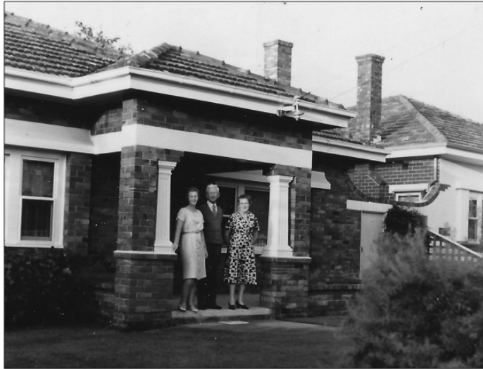
Fig. 4. Front garden at 35 Kent Road, 1960s. The porch with its square pilasters, and the cream brickwork across the façade, exemplifies the ‘featurism’ decried by Robin Boyd in The Australian Ugliness (1960).
