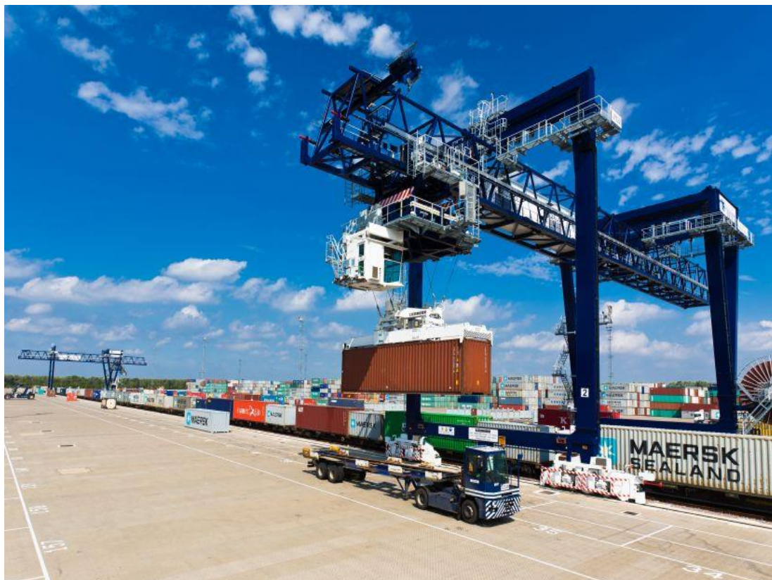
Figure 3.3: RMG in operation, (Source, Port of Felixstowe)
