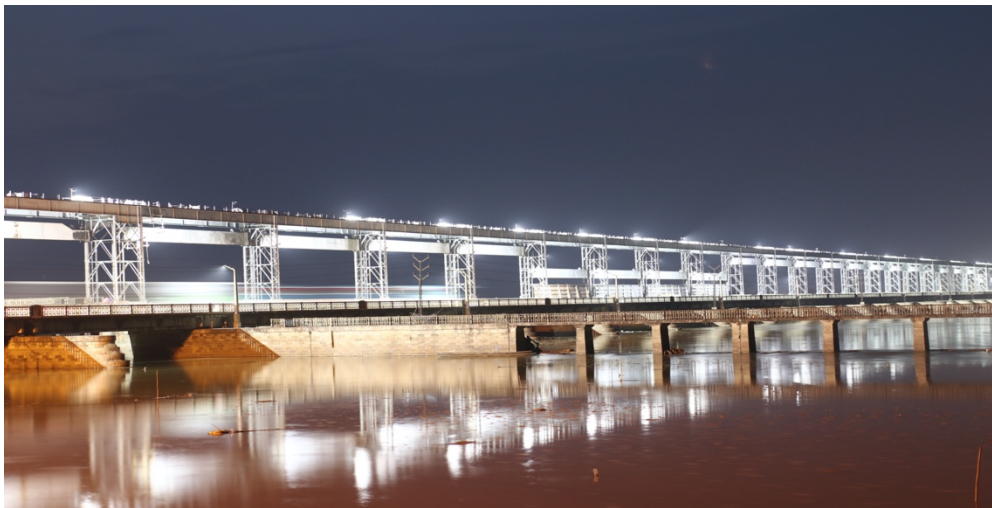
Photo 1: Koshi Barrage, Nepal
