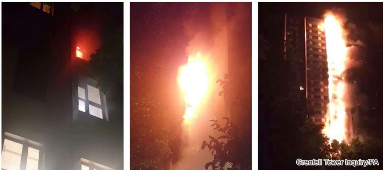
Figure 74: Images of the Grenfell Tower fire taken on mobile phones.
