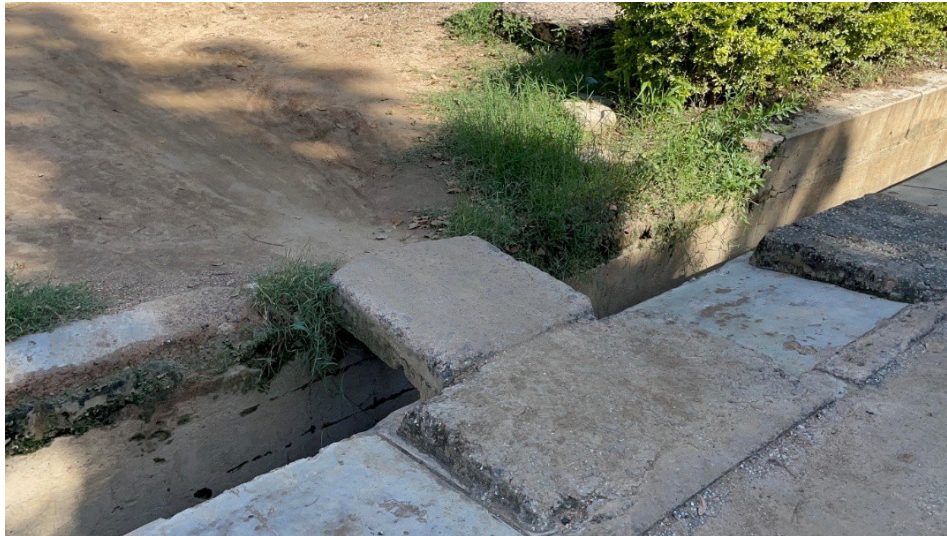
Image 3: A drainage ditch with a single concrete slab on top
