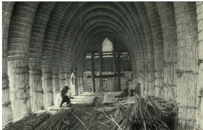
Figure 10: A mudhif during construction (Thesiger, 1964)
