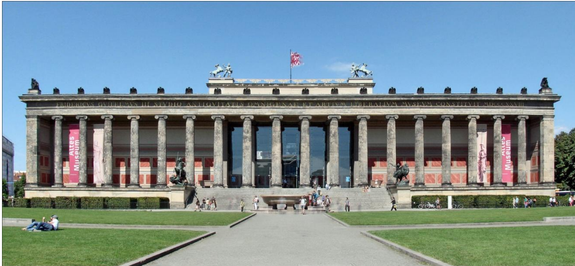
Figure 2.4 Recent photograph of the Königliches Museum (Altes Museum), Berlin. Architect Karl Frederick Schinkel. Constructed between 1816 and 1828. Credit: public domain.
