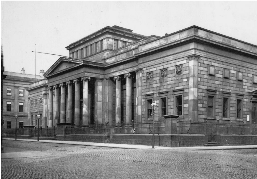
Figure 2.12 Photograph of the RMI Building, G. Grundy, 1861. Manchester Central Library GB127, M59060.
