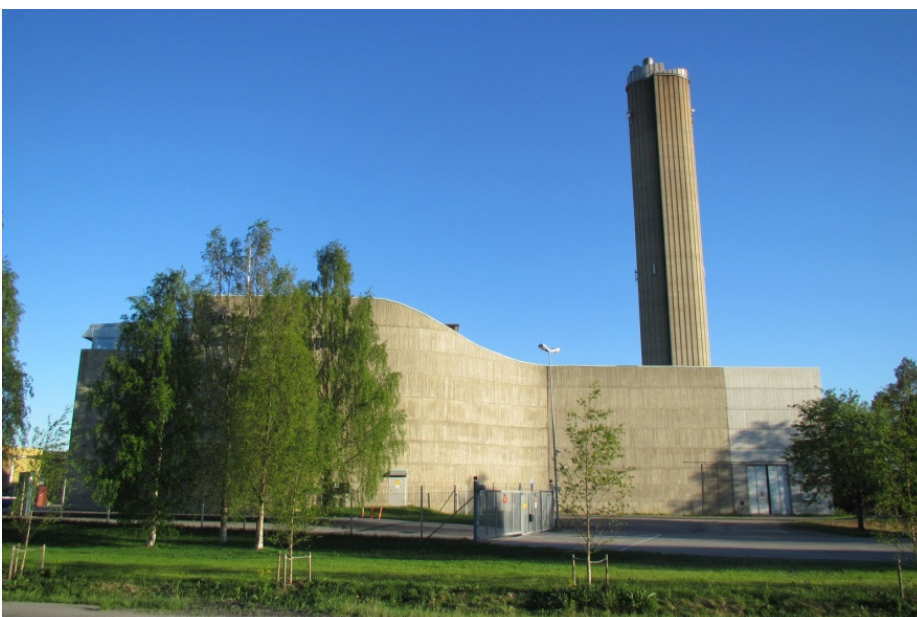
Image 6: Incineration plant in Umeå
